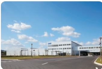
New building of Tanabe Plant
